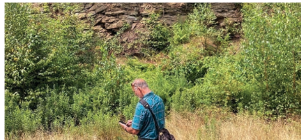
Abandoned mine land highwall investigation
