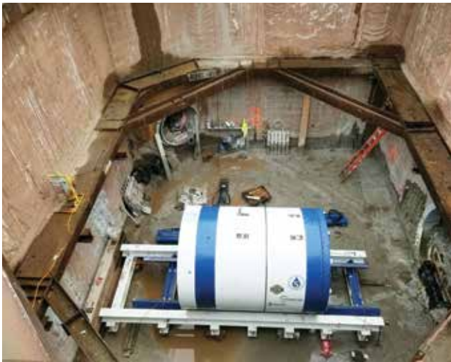
Figure 6 – 96-inch MTBM awaiting the start of tunneling
