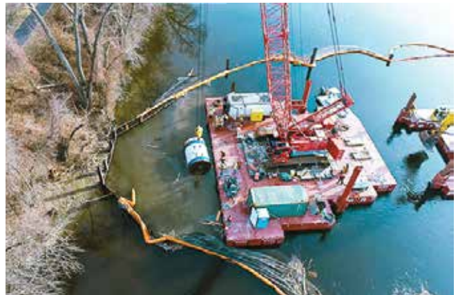
Figure 7 - Retrieval of the 96-inch MTBM from the Connecticut River
