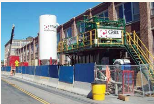
Maintaining 2-way traffic in tight urban setting for microtunneling on East Boston Branch Sewer
