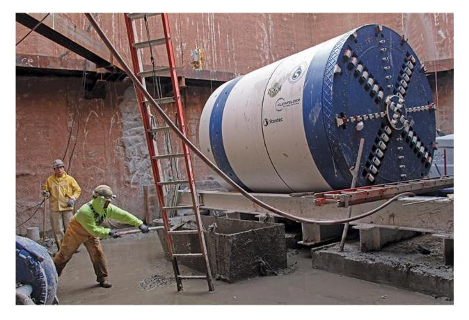
The project team extended the length of the tunnels so the microtunnel boring machine could drill through the riverbed slope underwater without need for a receiving pit.
