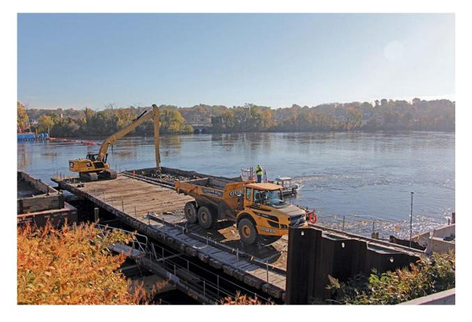
Crews hauled dredged material across the river by barge for removal and temporary storage on site.
