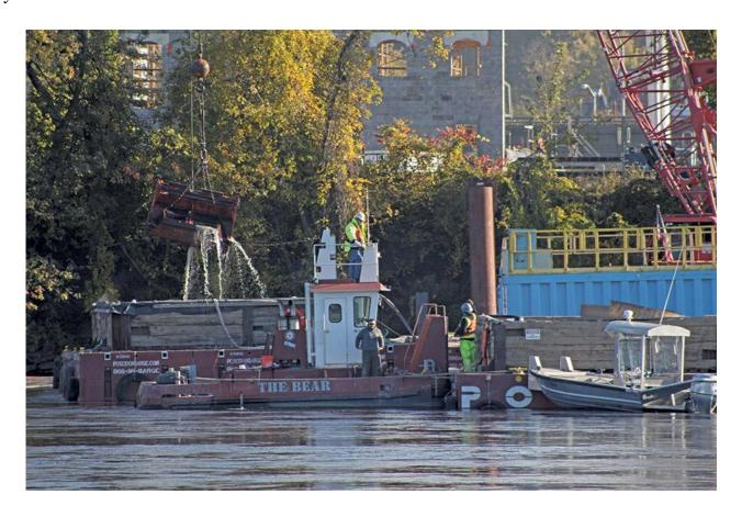
The project's dredging operation began excavating the 59-ft-wide by 15-ft-deep trench from the east side of the river working toward the west for the pipelines from the pump station to the treatment facility in December 2021.
