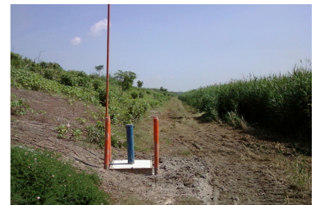
Inclinometers monitor slope movement
