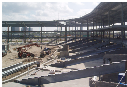
Structural steel observation was conducted
