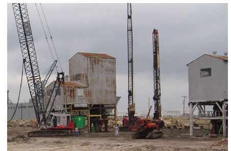
Industrial heritage was preserved
