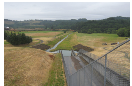
Spillway chute walls
