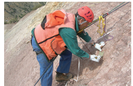
Rope-access inspection of rock cut
