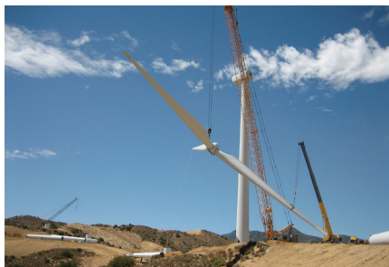
Hoisting wind turbine blades
