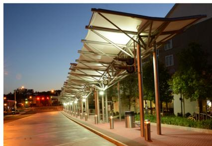
Stainless steel frame tension fabric structure
