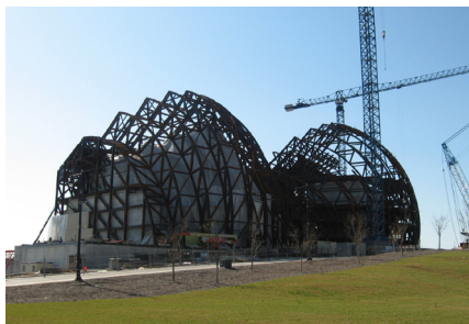
Structural steel frame
