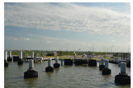
Ferry landing area
