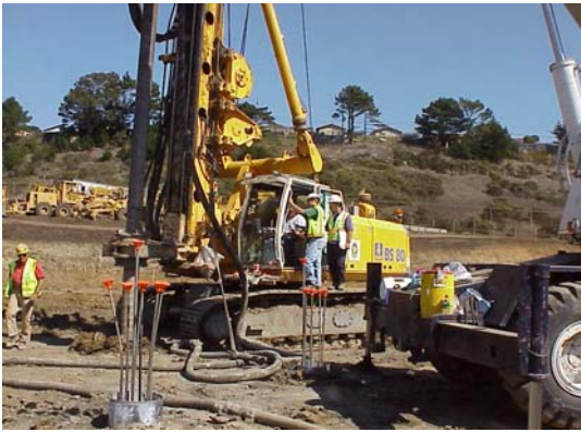
Photograph 3 – APDG Pile Installation
