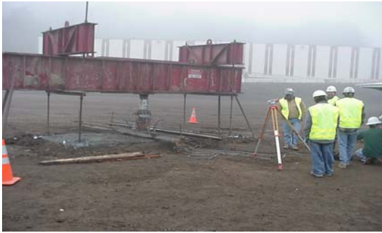
Photograph 1 – Load Test Set-Up
