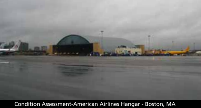
Condition Assessment-American Airlines Hangar - Boston, MA
