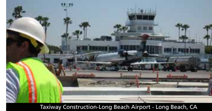
Taxiway Construction-Long Beach Airport - Long Beach, CA
