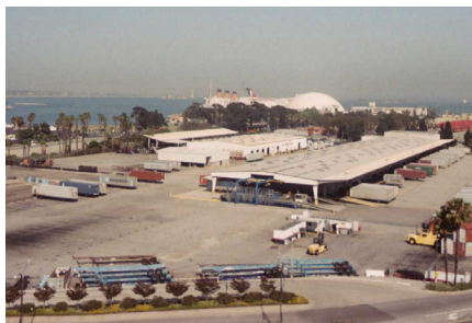
Site conditions prior demolition
