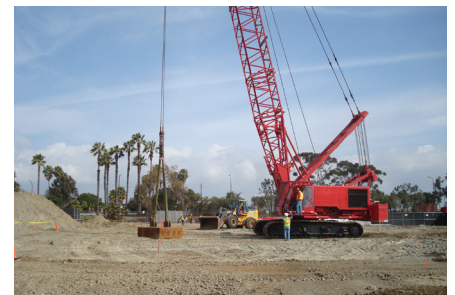
Deep dynamic compaction rig
