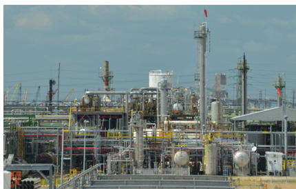
Chemical plant facility
