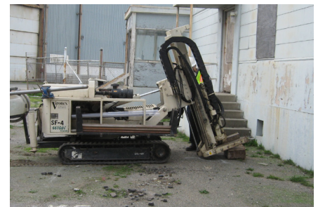
Direct push angle boring
